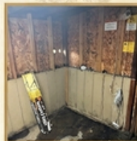
Rear Storage Area
